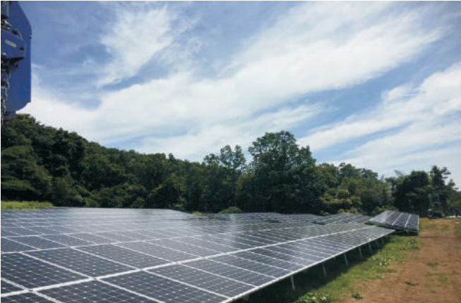
Hyogo and Tanba City 1.7MW Bottom Lock
