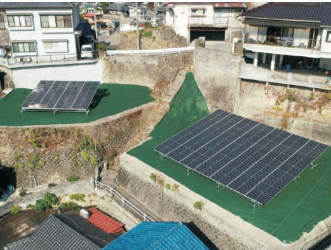
Genshima Dingwu City Single Pipe Foundation
